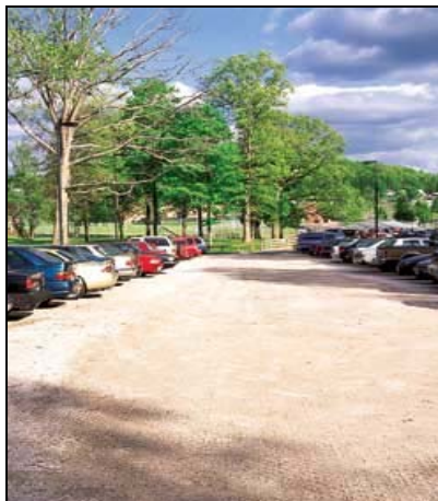
An example of porous paving (photo from Landscape-Online.com)
