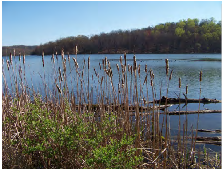
WASHINGTON DAM #4, North Franklin Township
